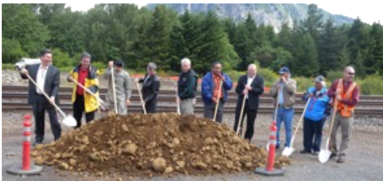
Tribal, CRITFC, U.S. Corps of Engineers, BIA, and Oregon State Parks representatives turning the first spadeful of earth to mark the beginning of construction of the Wyeth Treaty Fishing Access Site.
