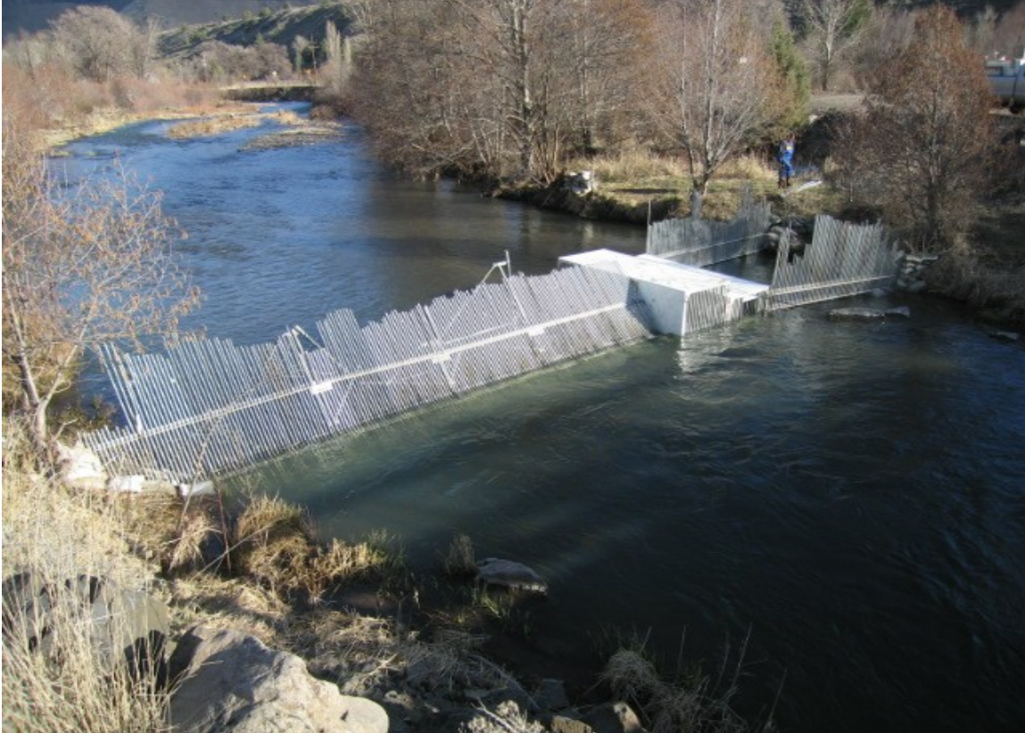
Figure 7. Photograph of the picket weir operating on Shitike Creek in 2006
