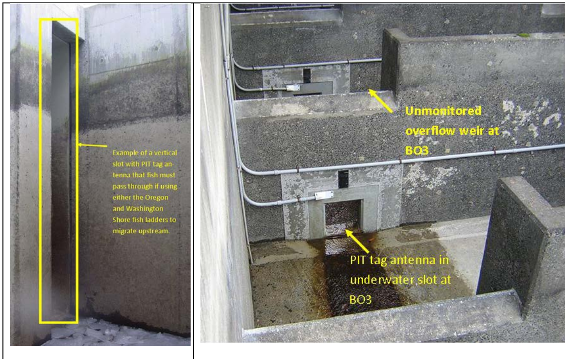
Figure 4. Photos of the two types of PIT tag antennas at Bonneville Dam. The vertical slot antennas are at the upper end of both ladders, while the underwater antennas are in the lower parts of the ladders (photos courtesy of PTAGIS).
